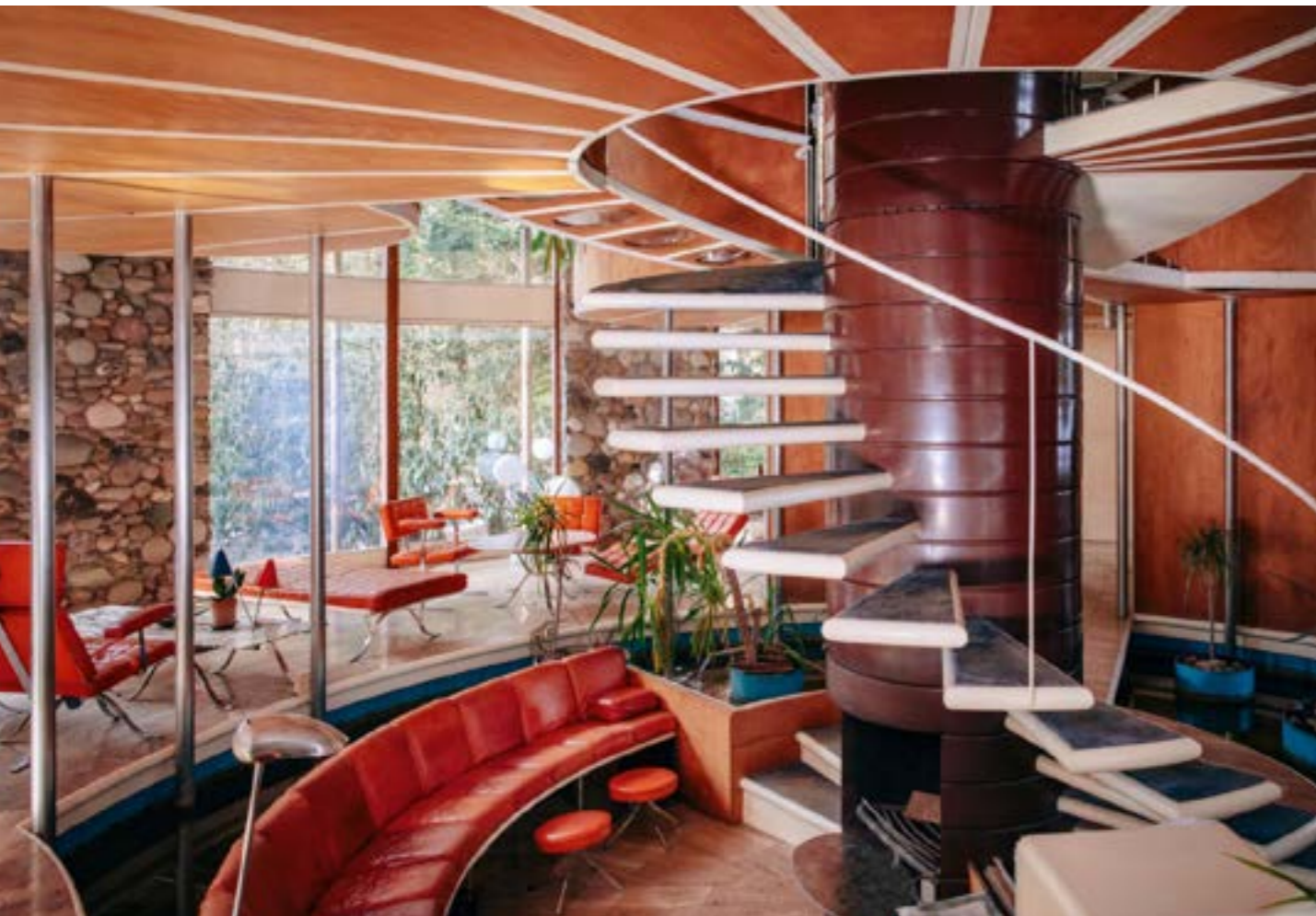
The steel spiral staircase forms the main core of the building. It is one of Otto Kolb’s most important inventions
