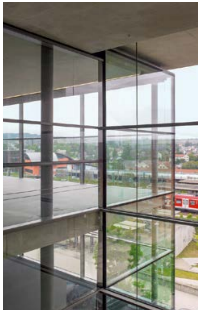
Clear corner: the distinctive corner in the glass facade showcases some of the company's core values – depth, diligence and openness
